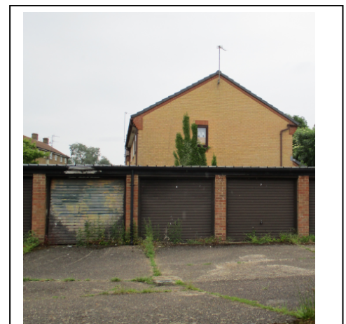
Image: Badly designed parking – isolated garage courts are often unused and accommodate anti-social behaviour and crime
